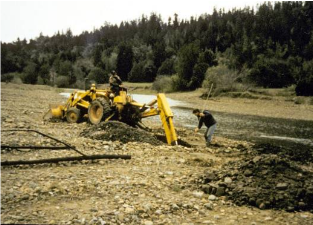
Figure 20. This photo shows Chris Tebbutt deep planting cottonwood and willows in 1984. The dark branches at the left are fence post-sized black willows. Photo by Chris Tebbutt.
